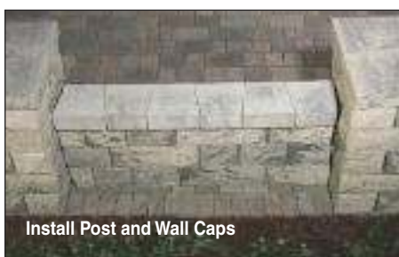
Finish wall panel to desired height.
