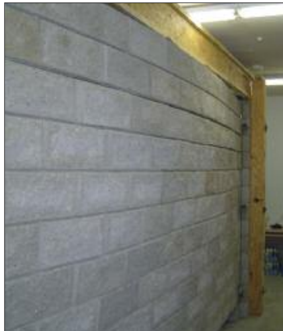
Flexing panel with Intermediate Column
