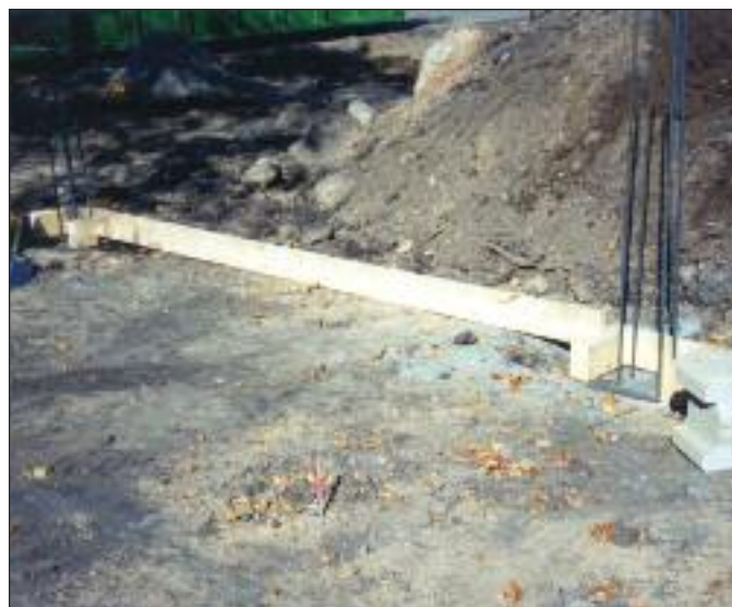
Figure 1: AB Fence Pile Layout Jig
