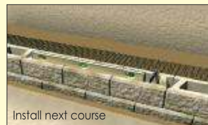
Install AB Reinforcement Grid
