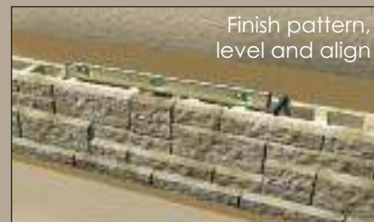
Compact on block and behind
