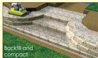
Install wall out from stairs
