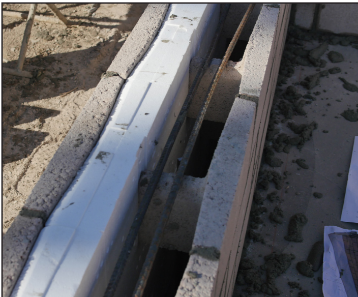
Hi-R H units are suitable for construction of bond beams without the need for any modifications to the units and the insulation inserts remain fully in place
