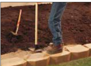
2. Place & Compact Backfill
