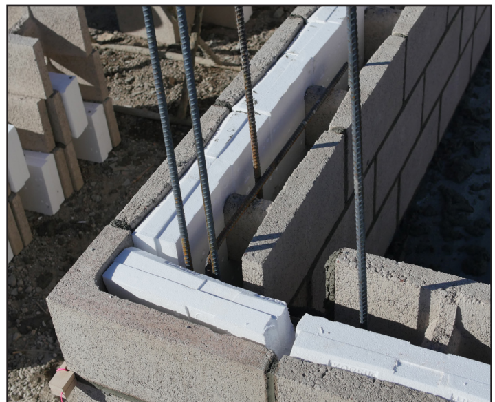
Insulated corners are built using conventional masonry fittings and Hi-R H units
